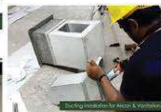
Ducting Installation for A/C & Ventilation
